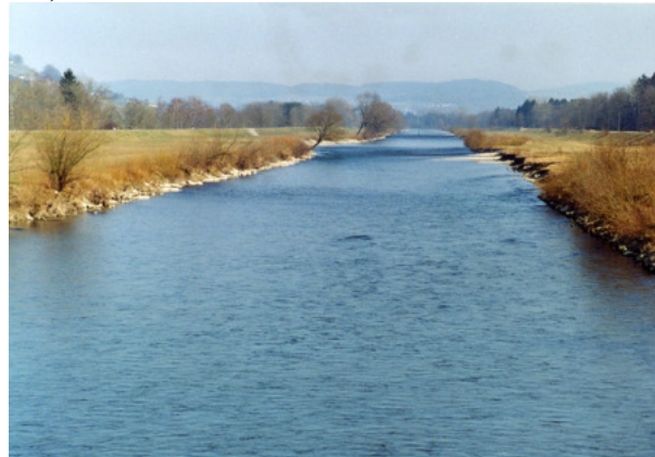
Tailwater: Trapezoidal profile with forelands and a small widening.
