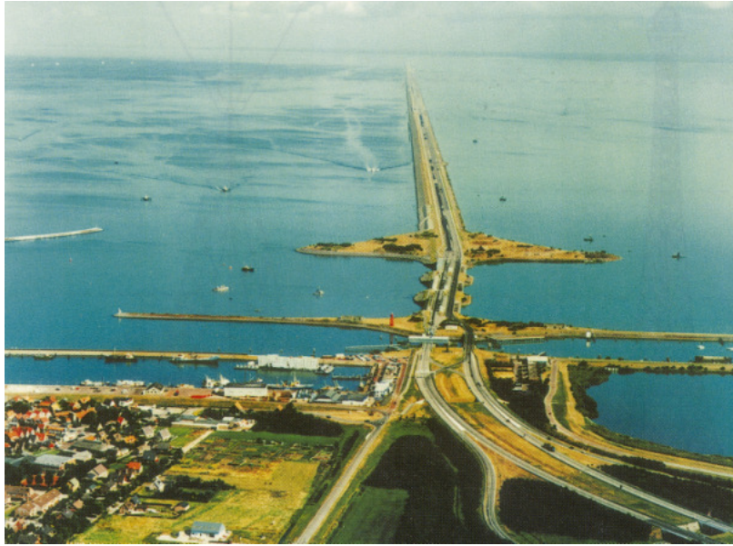
Fig. 13: The 32 km long main dam separates the Wadden Sea from the fresh water of Lake IJssel (IHP / OHP 1996: 94)
