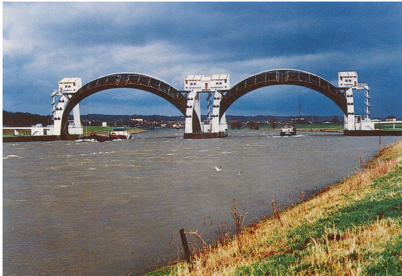
Fig. 12: The weir at Driel in the Lower Rhine. The weir directs water to the north or allows it to pass on to the west of the country (IHP / OHP 1996: 94)
