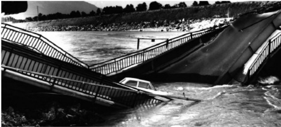
Fig. 94: The bridge Buchs-Schaan collapsed in 1972 because of the erosion of the river bed. After the collapse numerous bed load excavations were stopped (Landesarchiv Vaduz) (Zarn 2005)
