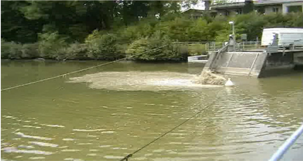
Fig. 45: Sediment laden water release in front of power intake (De Cesare et al 2008a)
