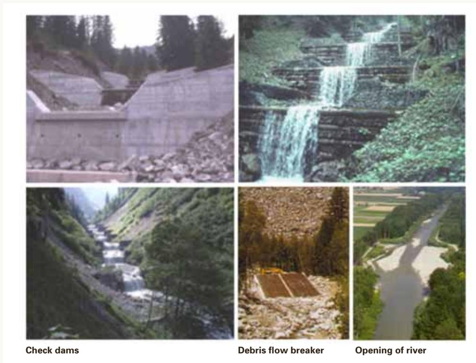
Figure 1.3 Stabilisation of torrents by check dams, debris flow breaker and river opening
