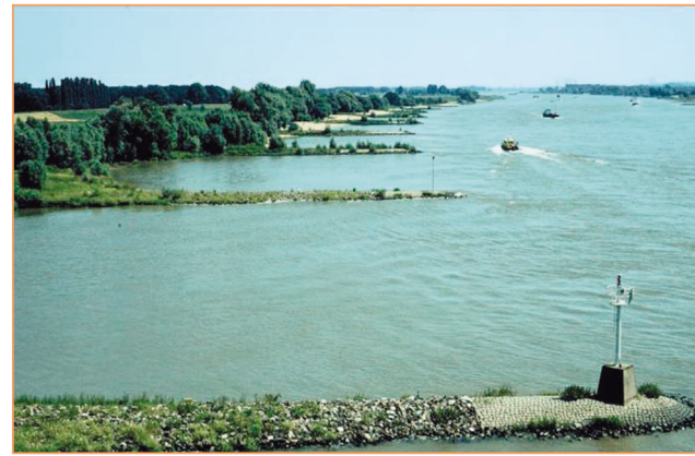
Fig. 2 Groyne fields in the river Waal (Netherlands)
